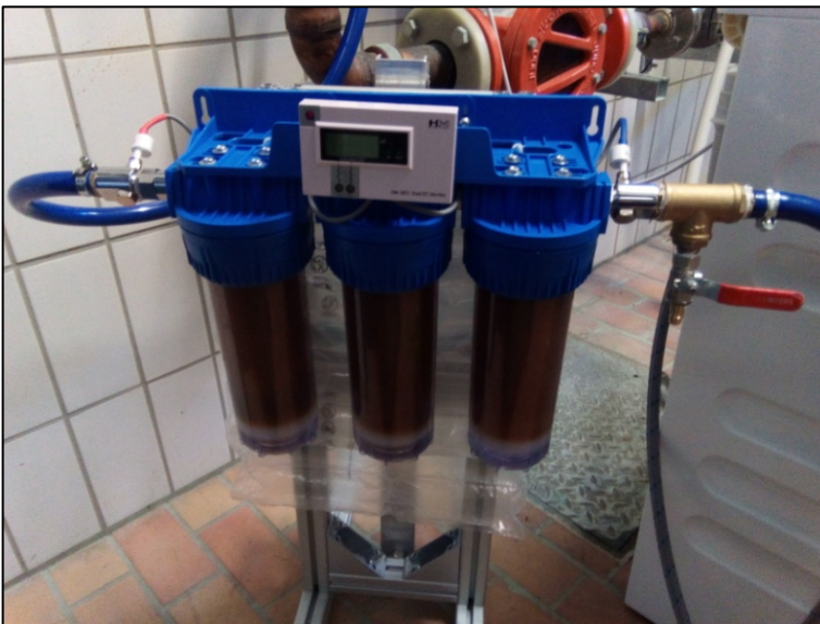
Figure 8: Demineralizer AFT Pro with conductivity measurement and filling tap (test operation)
