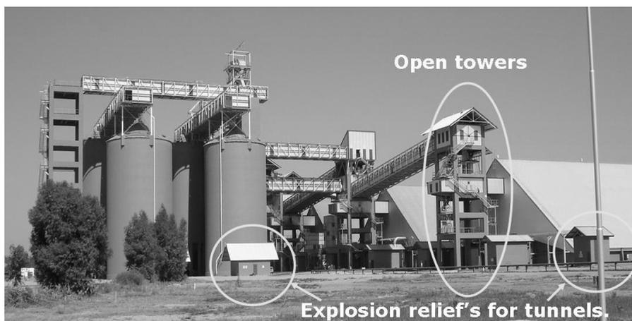
**Figure 6** Open towers and explosion reliefs for tunnels.
