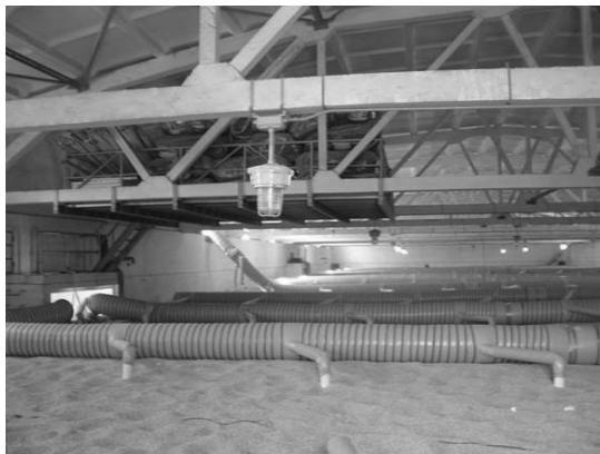
Figure 4 Ventilation system vertical aerator pipes spaced in grain
