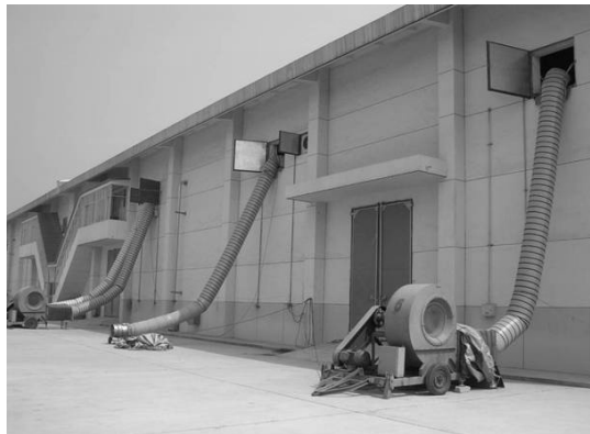
Figure 3 Combined vertical ventilation system blowers and air supply hoses
