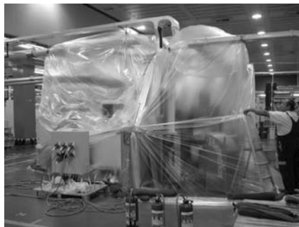
Fig. 6 Spot heat treatment
